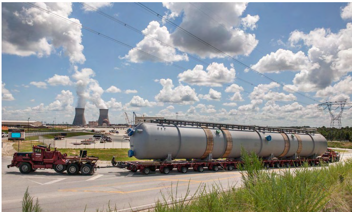
"Equipment arrives at Vogtle nuclear plant – August 2013" by NRCgov Courtesy of Georgia Power Company ©. (August 2013)
