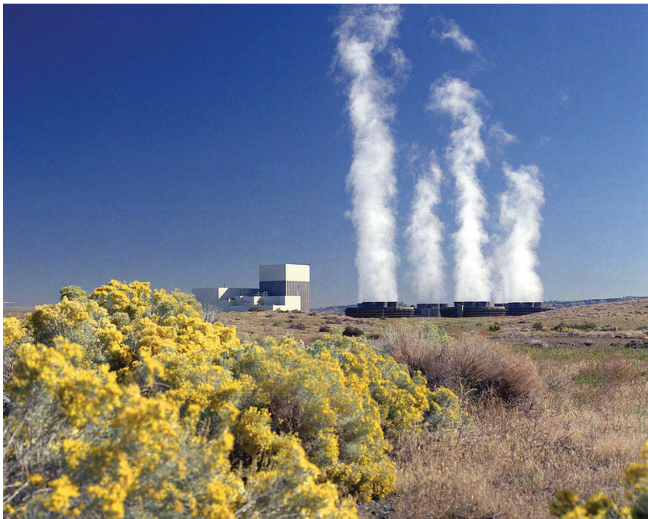
The Columbia Generating Station in Washington state, where X-Energy plans to demonstrate its Xe-100 reactor. "Columbia Generating Station, Unit 2" by NRCgov under CC
