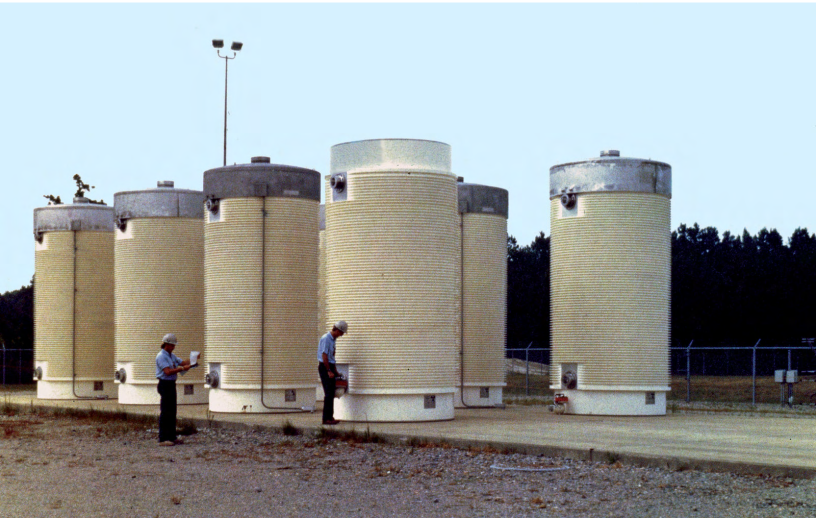
Inspecting a dry cask storage facility (Image Credit: US NRC )
