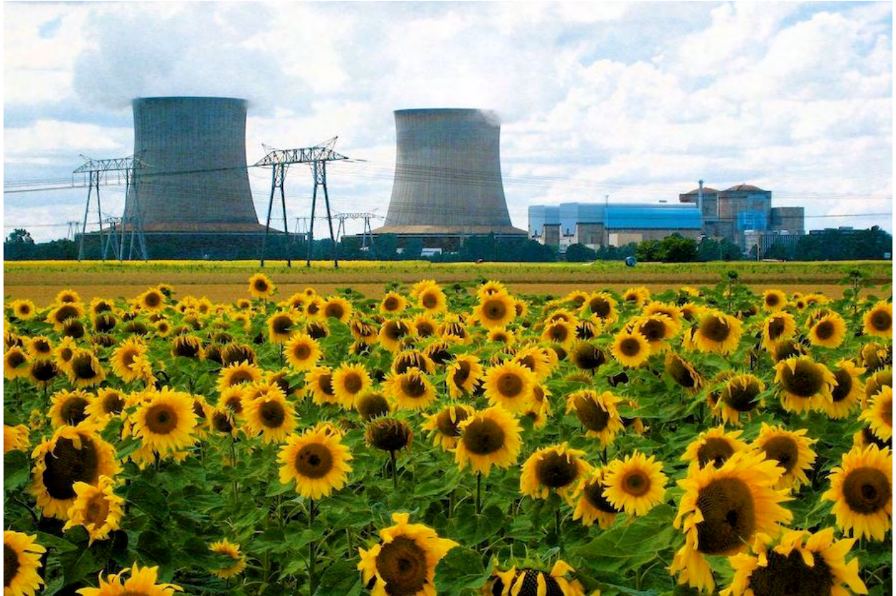
The Saint-Laurent Nuclear Power Plant in France, by Nitot under CC
